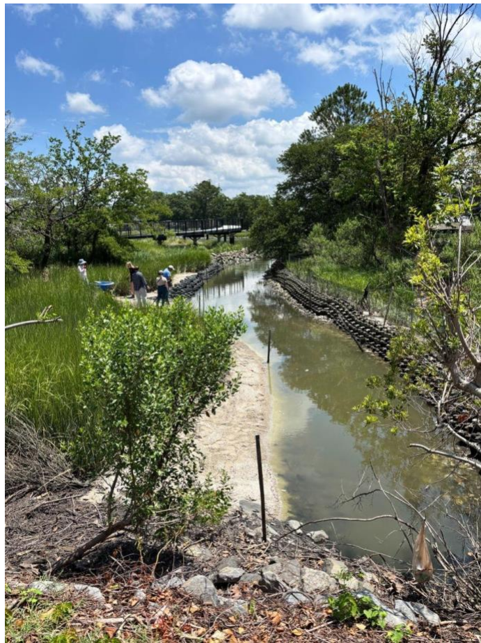
Figure 5. Restoration project using oyster castles along Knitting Mill Creek in Norfolk, VA. Photo credit: Laura Costadone.
