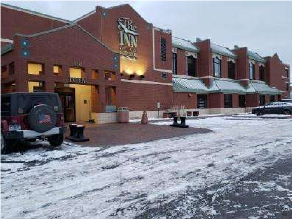
Figure 44. Heated Pavement: Entryway
