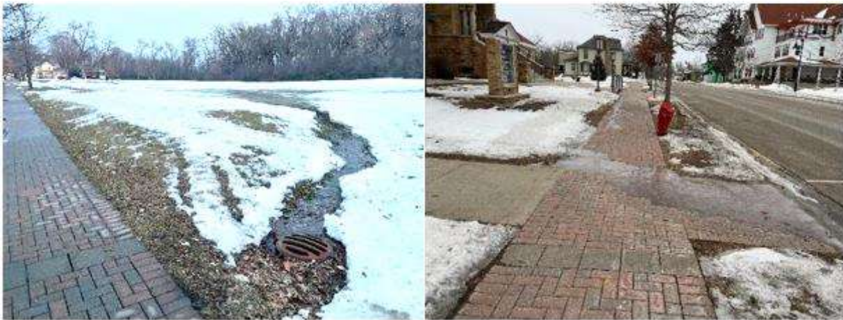
Figure 15. Horizontal Drainage: Low vs. High Salt Design
