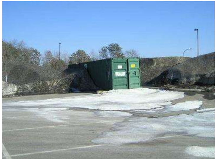
Figure 40. Salt Storage: Good Containment, Poor Location, Poor Housekeeping
