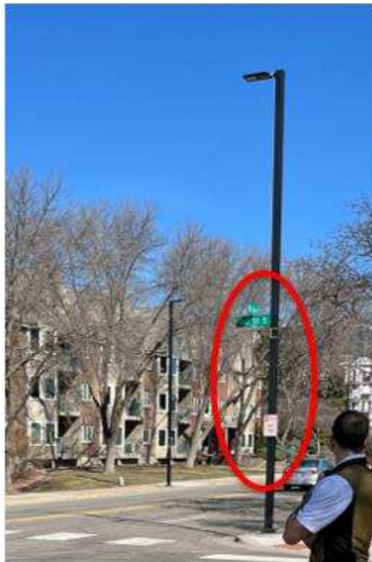
Figure 24. Reduction of Plow Obstacles by Combining Light Post, Street Sign, and Parking Notice
