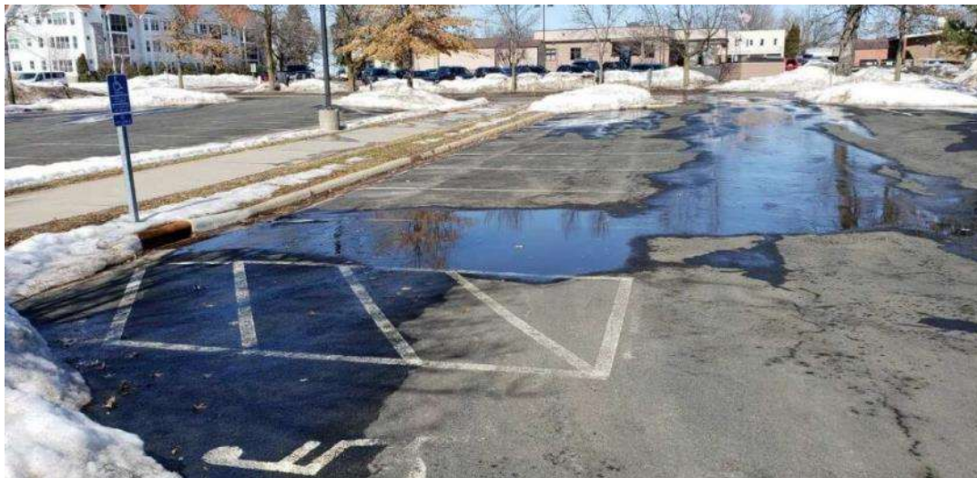
Figure 28. Meltwater Sprawl from Snow Storage, soon a Sheet of Ice
