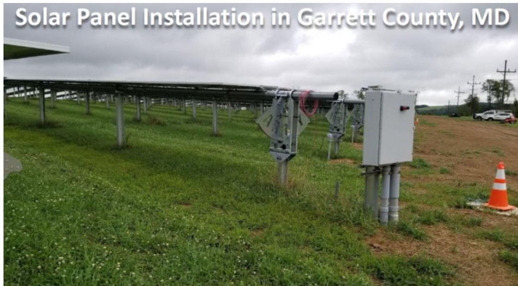
Figure 7. Solar panel installation in Garrett County, Maryland.
