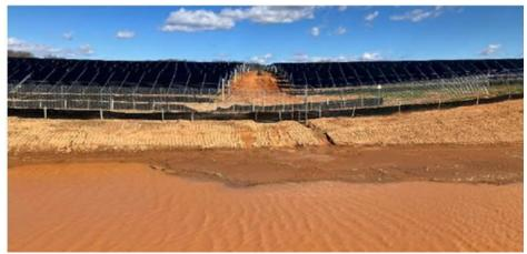
**Figure 6.** Site under active USS development in Virginia before mandatory stabilization and revegetation within 7 days of achieving Final Grade. Final Grade is normally achieved before solar panel installation - but DEQ often sees this requirement ignored resulting in the conditions shown in this photograph.
