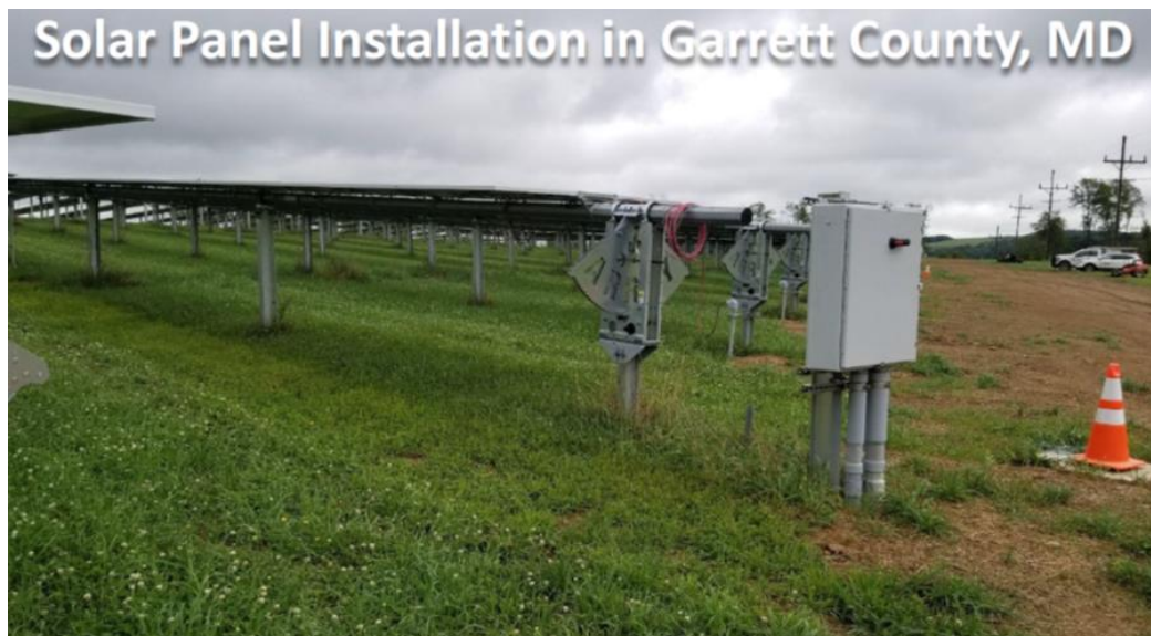
Figure 7. Solar panel installation in Garrett County, Maryland.
