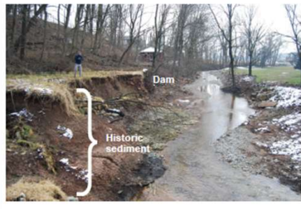
Figure 1 Erosion of legacy sediment following breach of Strobers Dam in Pennsylvania in 2011. Bank sediments are upstream of the breached dam, and the top of the bank matches the top of the dam.
