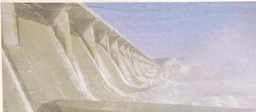
Conowingo was built in 1928 to generate electricity, and it inadvertently acted as a trap for nutrient and sediment pollution flowing downstream to the Chesapeake Bay. Over the years, sediment buildup behind the dam has reduced its pollution-trapping capacity. (Dave Harp)
