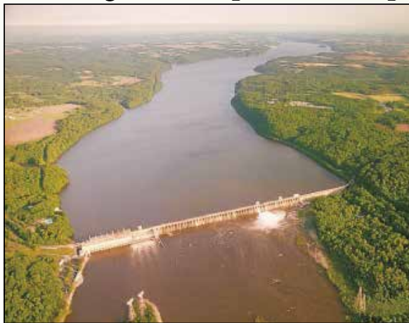
A report earlier this year cautioned that phosphorus and sediment discharges from Conowingo will likely increase in the future as the sediment storage capacity of the reservoir behind the dam nears its capacity. Photo / Dave Harp
