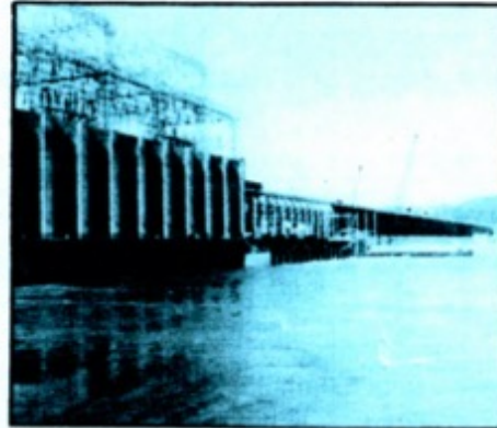
The Conowingo Dam is the largest dam on the Susquehanna, but its reservoir will be filled with sediment in 20 years.
