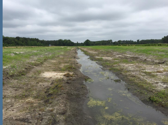
2-stage Ditch (Newly Constructed)
