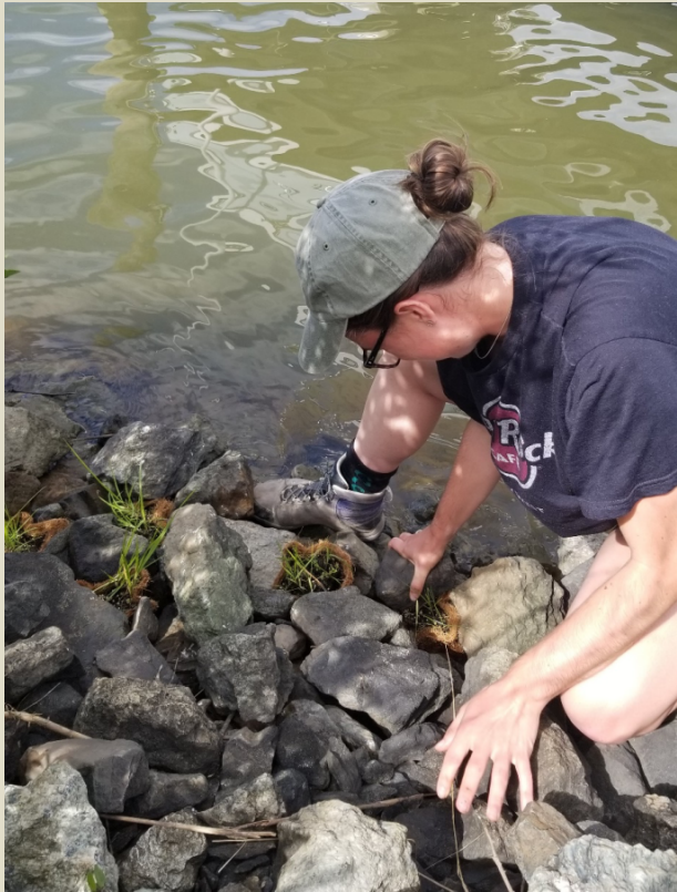
Above: a volunteer wedges a plant into the riprap.
