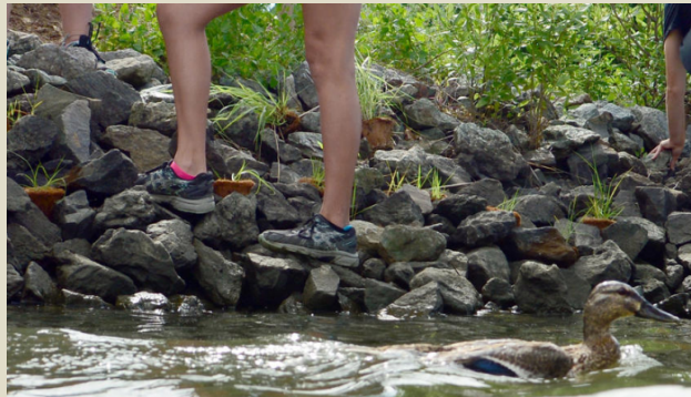
The grasses in the coconut fiber pots are planted by wedging them in the voids of the rock.
