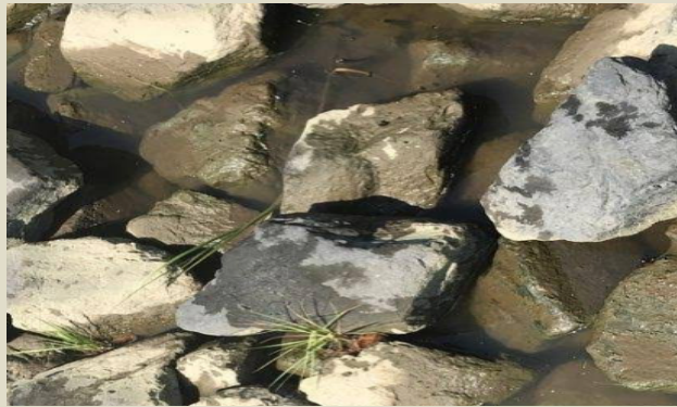
The grasses in the coconut fiber pots are planted by wedging them in the voids of the rock.
