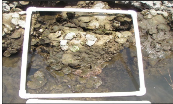
Breakwater- large quarry stone
