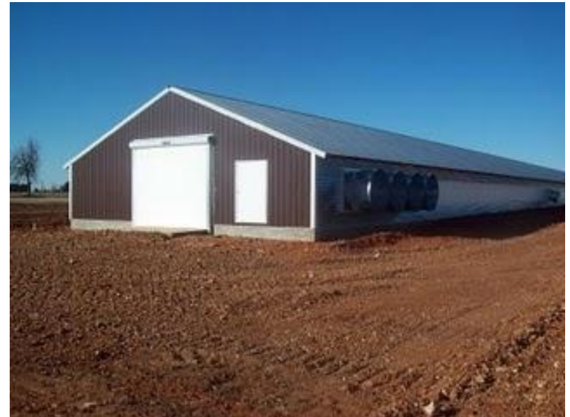
Tunnel ventilated poultry house
