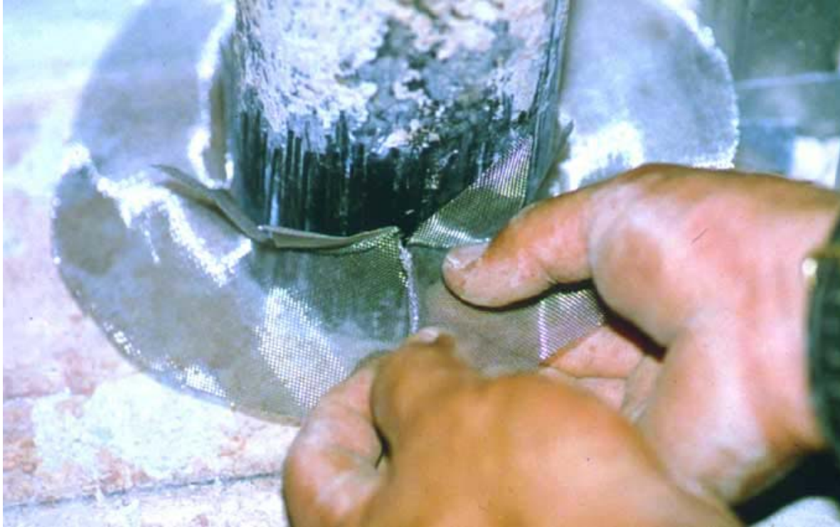
Installing TermiMesh (stainless steel screening)
