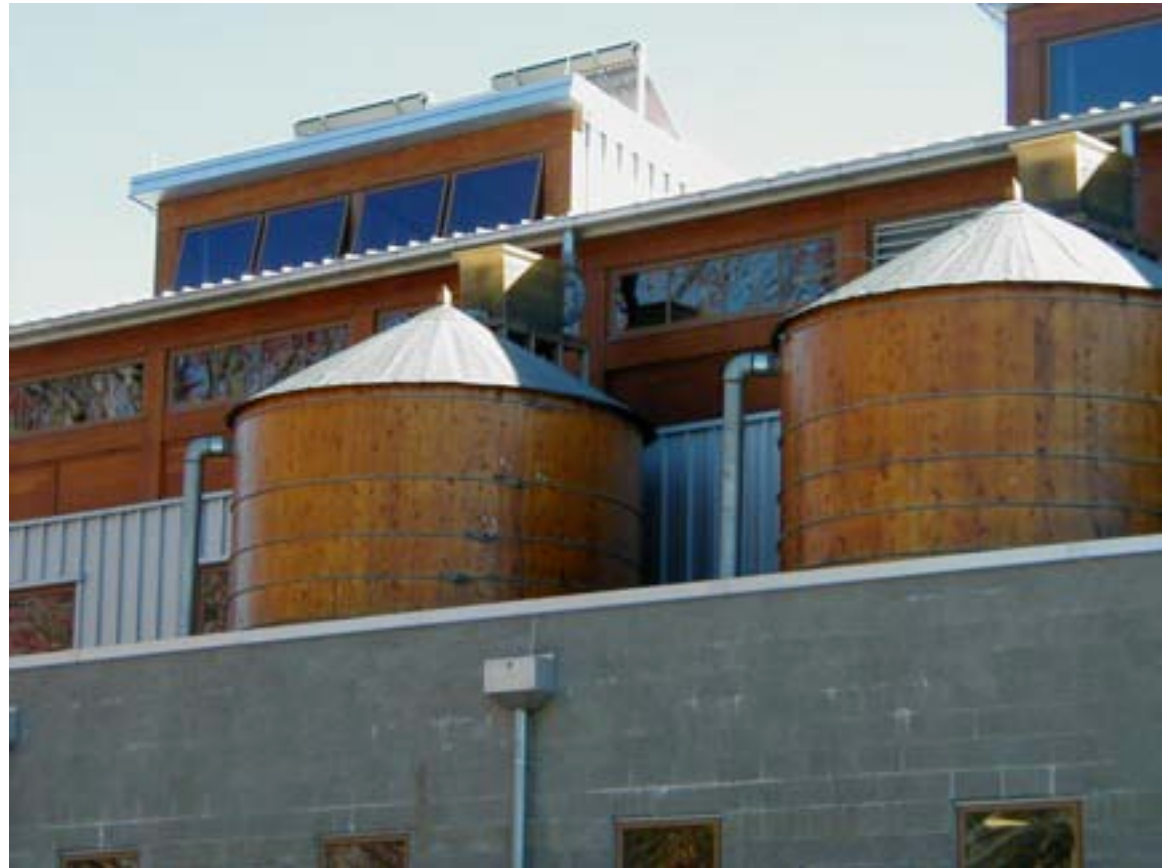
Rainwater tanks at the Chesapeake Bay Foundation
