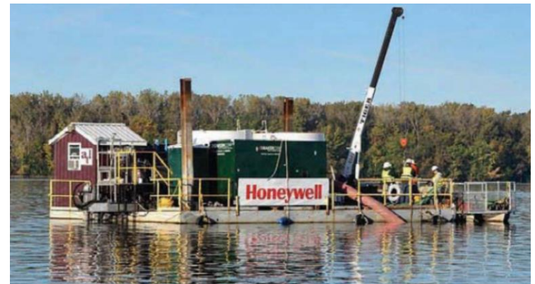
Whole lake nitrate addition for control of MeHg in Onondaga Lake. D. Mathews. Clean Waters, Winter 2017
