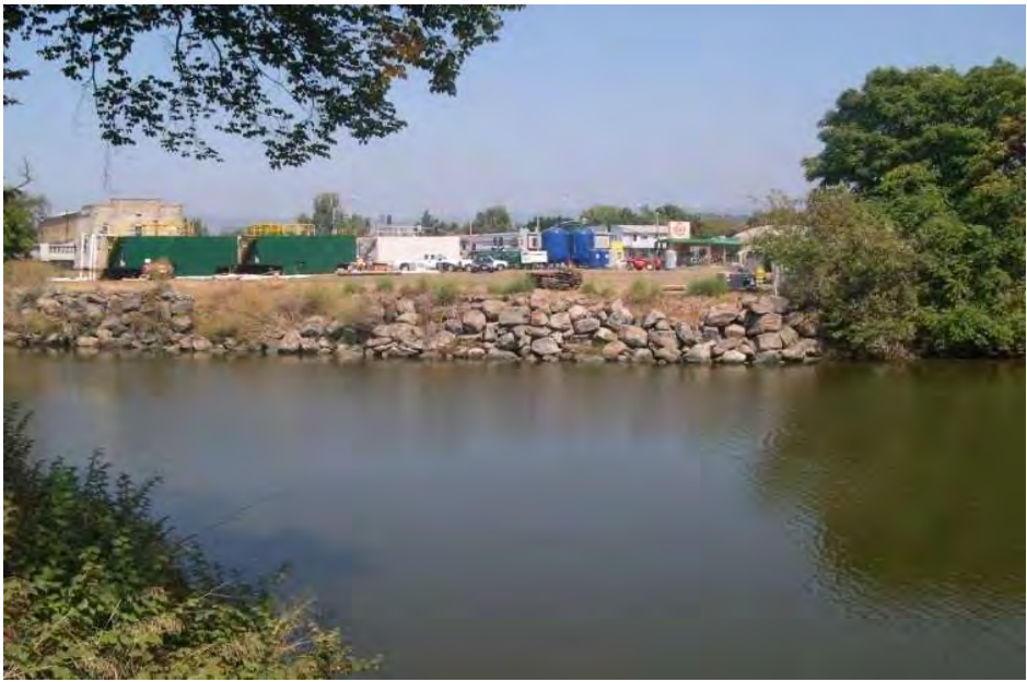
NAPA RIVER BANK BEFORE PROJECT
