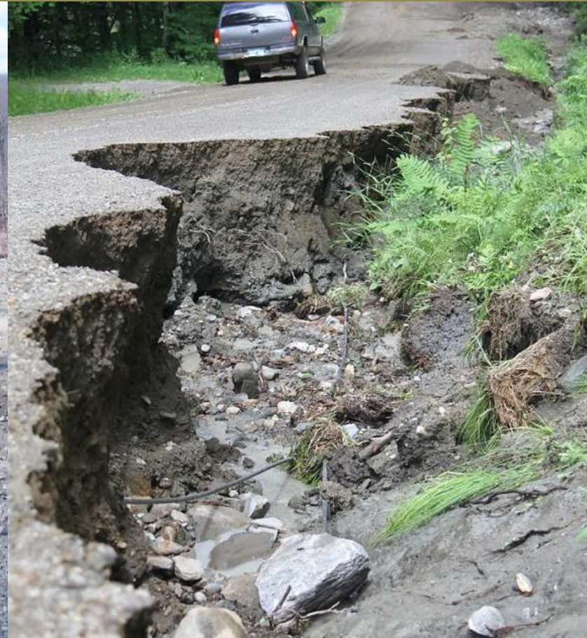
Storm-damaged gravel road
