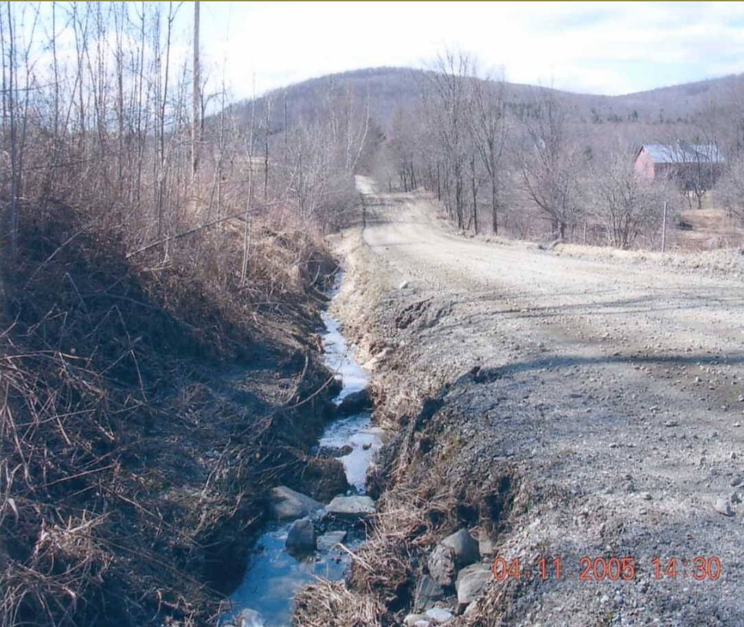
Eroding roadside ditch
