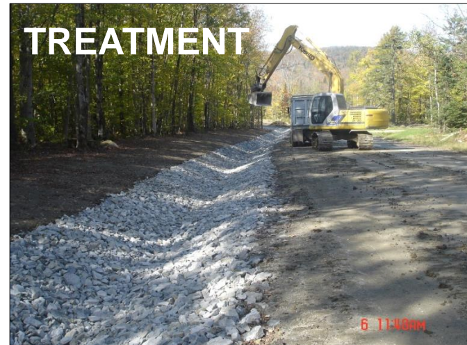
Ditch stabilization saves road and reduces erosion 27
