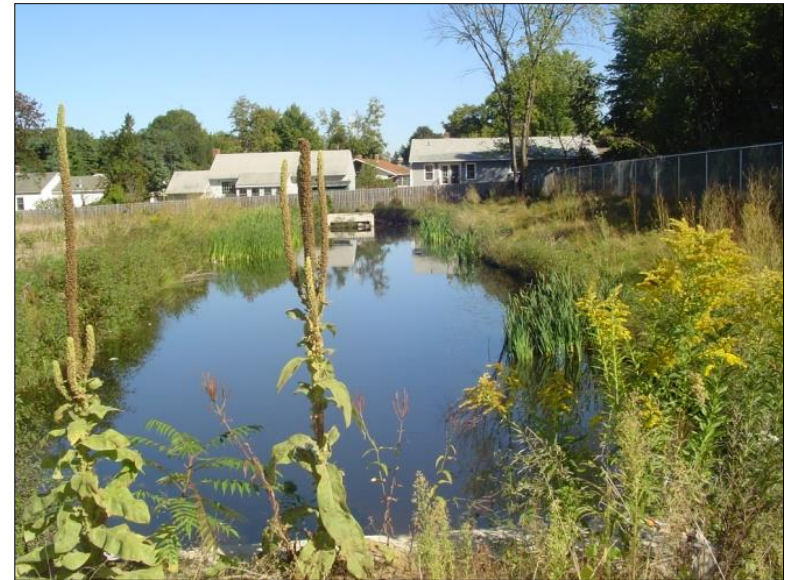
Expanded stormwater treatment pond
