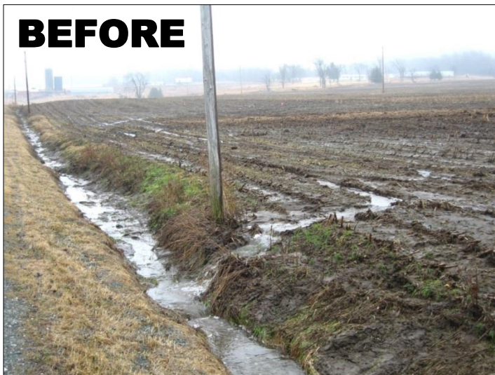
Runoff draining into ditch
