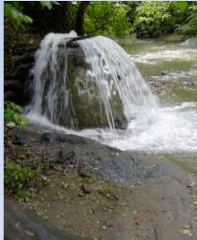
Surcharging sanitary sewer manhole, Gwynns Falls
