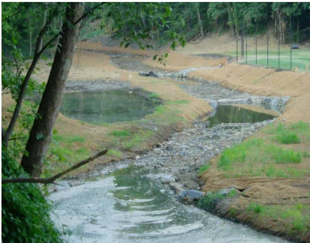
Constructed storm water wetlands
