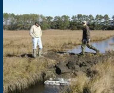
Targeted Wetland Restoration: Ditch Plugs
