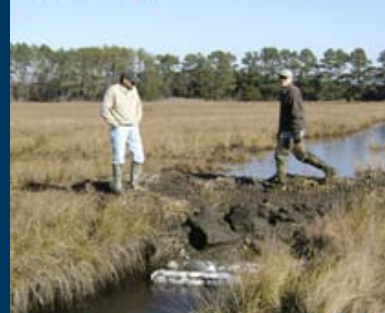
Targeted Wetland Restoration: Ditch Plugs
