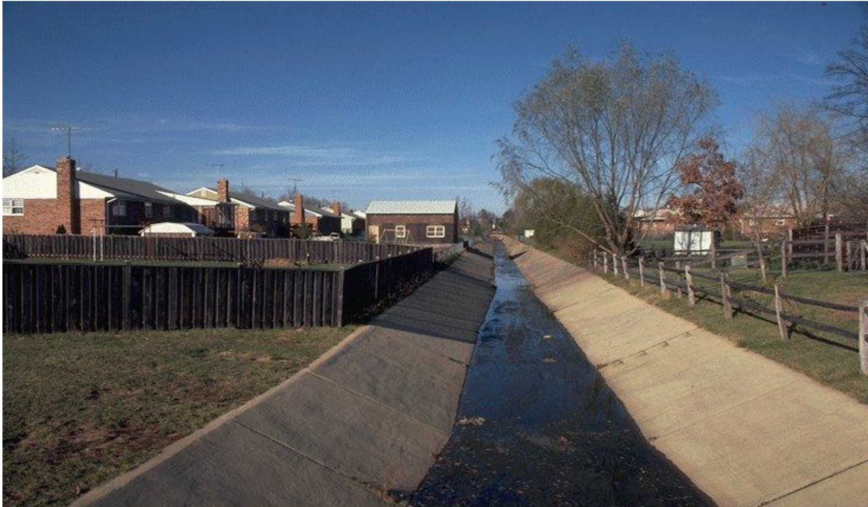
Fig. 3.10 – Stream channelization. Instream modifications, such as uniform cross section and armoring, result in ecological decline.
