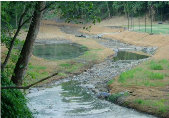
Constructed storm water wetlands
