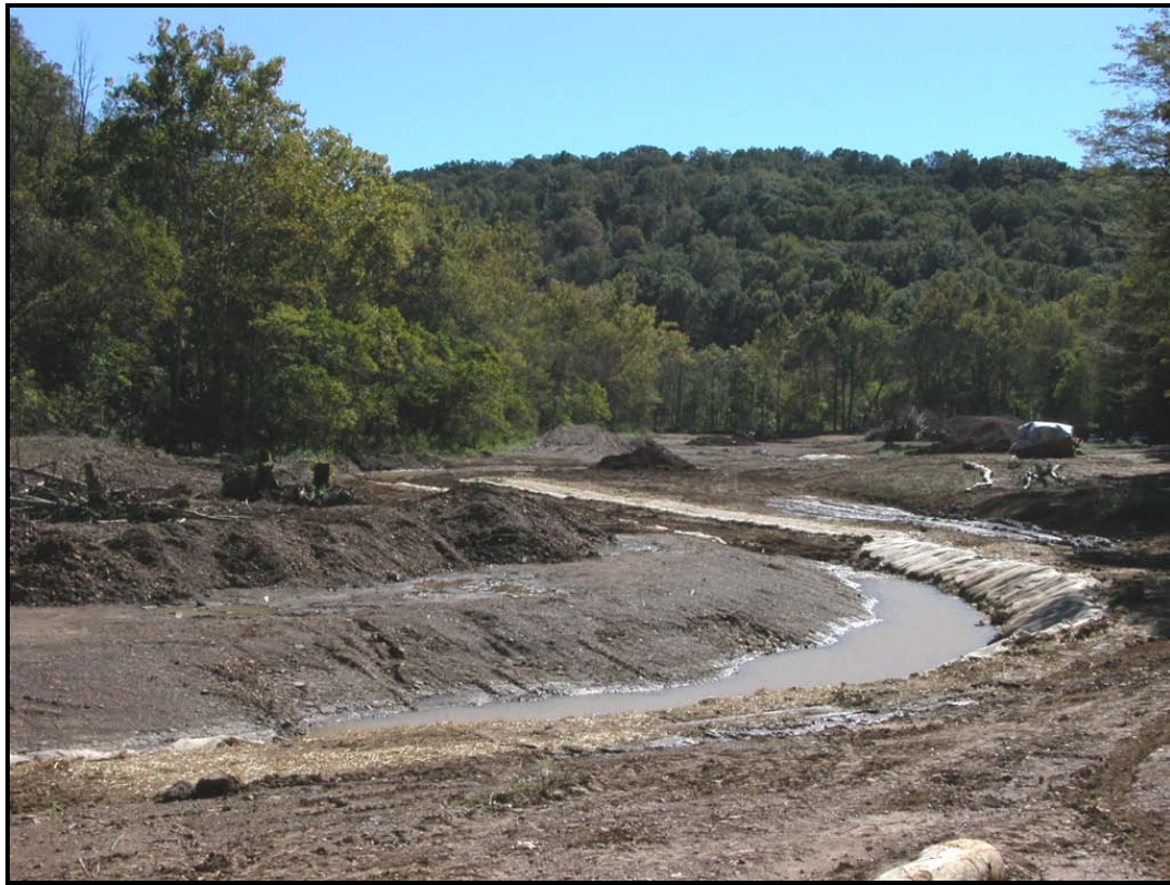
Left: Wilson Creek restoration in progress during summer 2003.
