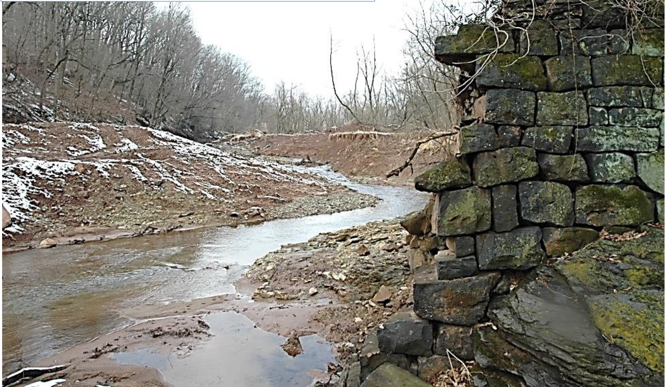
Indian Run, PA – Stobers Dam breach, 2011 Height 14 ft (4.3 m)
