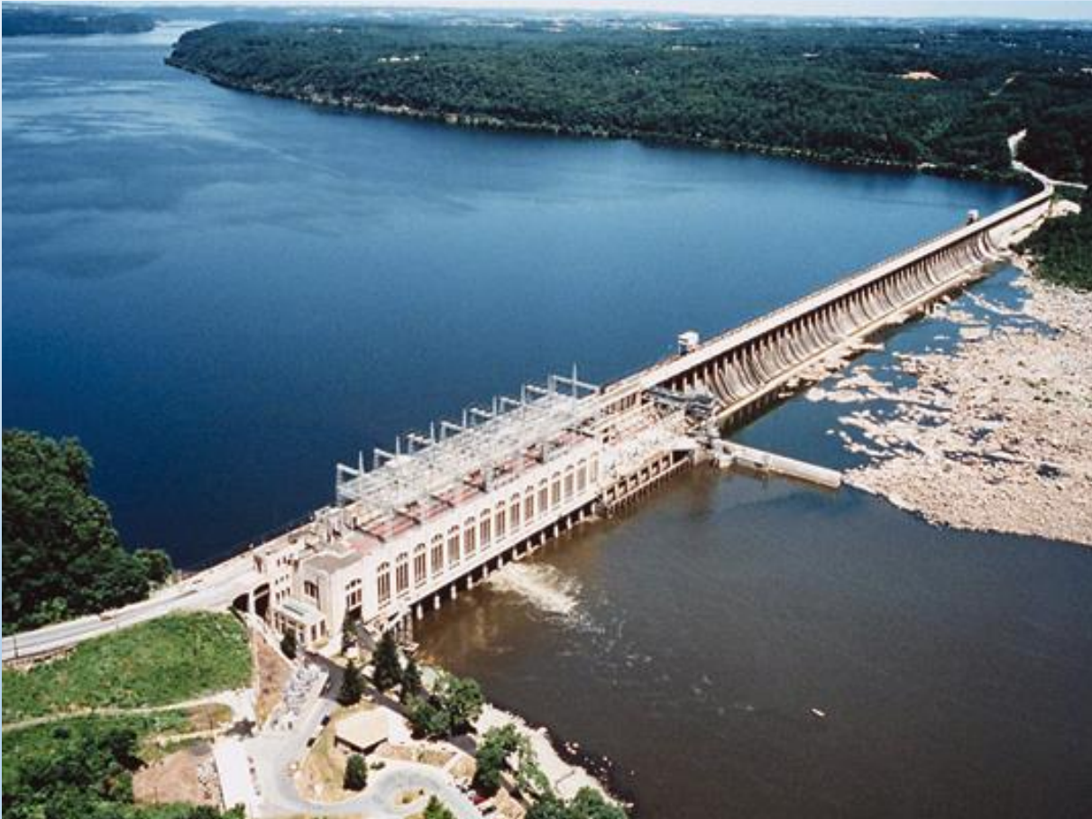
Photo of Conowingo Dam from www.chesapeakeboating.net
