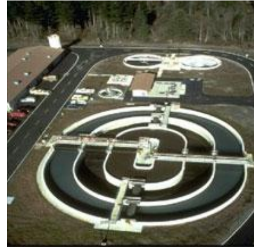
Orbal® Oxidation Ditch Source: Siemens
