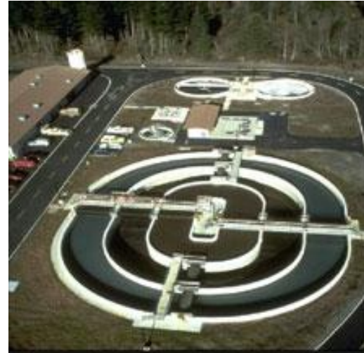
Orbal® Oxidation Ditch Source: Siemens
