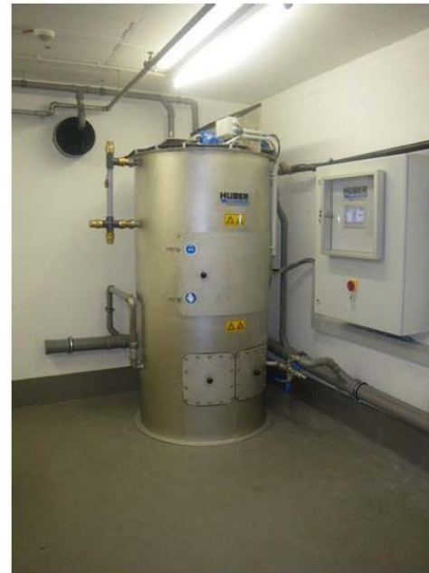
Figure 2-16 MAP (Struvite) Reactor at GTZ Headquarters (M.Winker, 2010). Reprinted with permission from GTZ.
